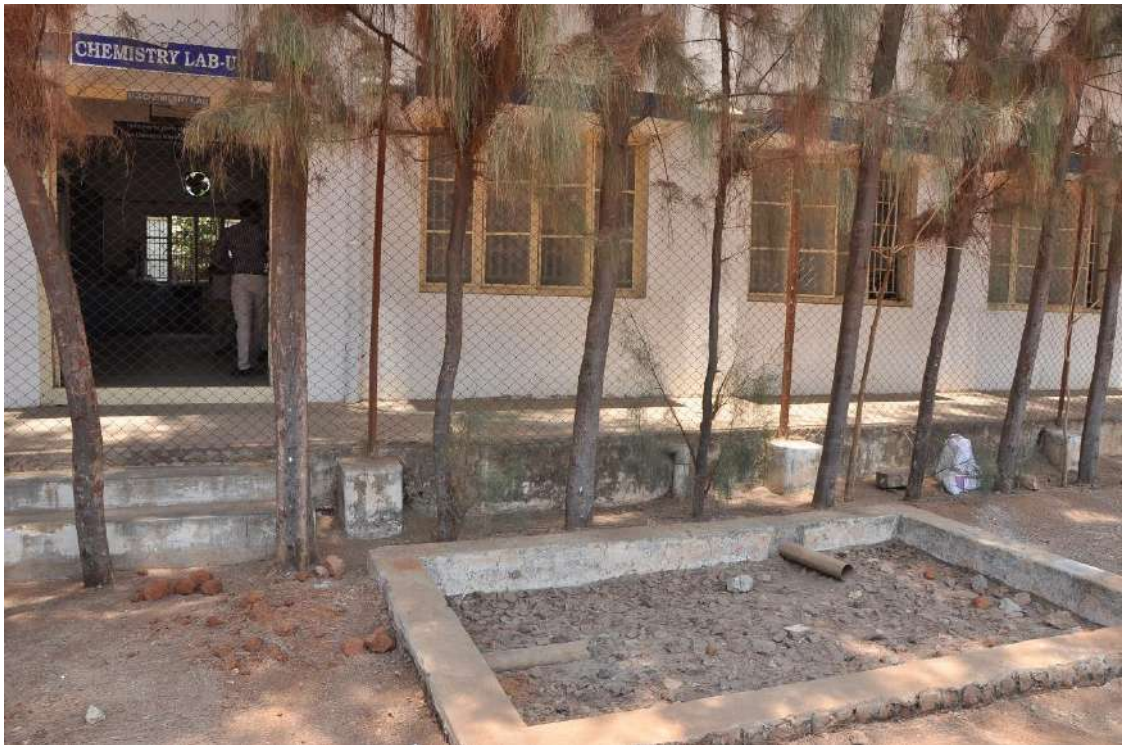
The rain water harvesting unit
