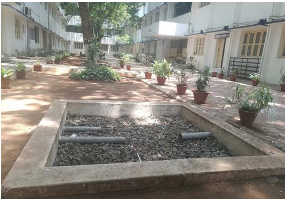
The rain water harvesting unit
