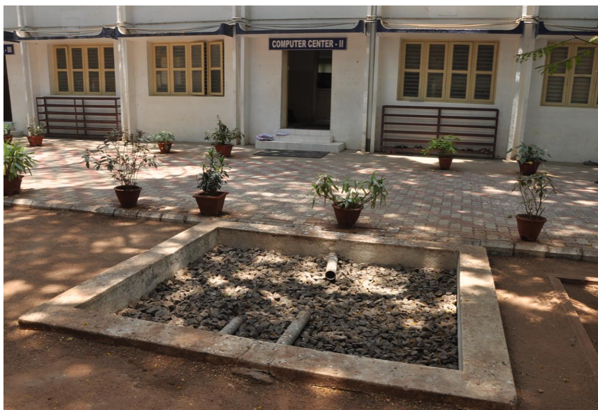
The rain water harvesting unit
